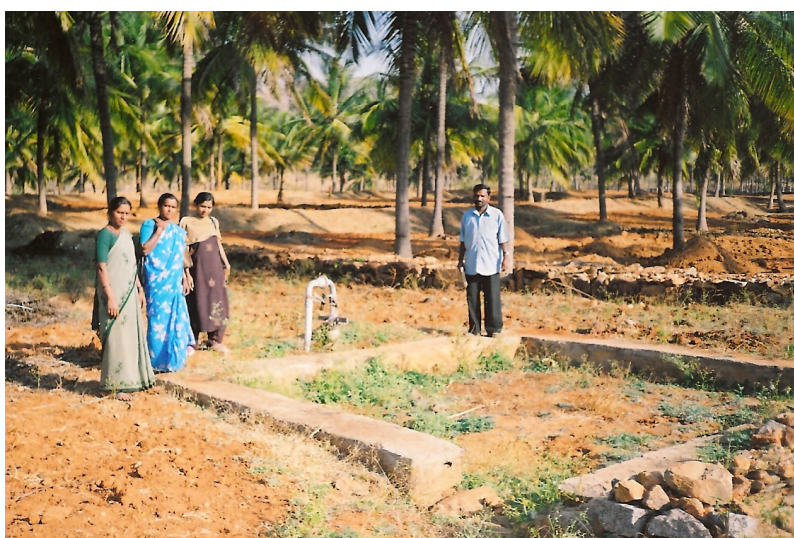
Fig 3: Recharge pit for irrigation borewell in Sujala watershed program
