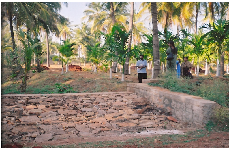
Fig 2 :Spillway constructed for runoff in the Sujala watershed, Karnatak
