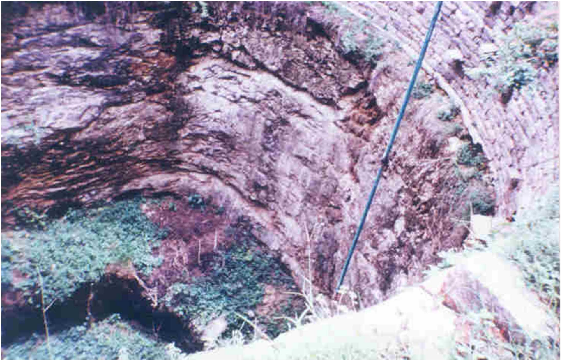
A failed well in Thippanahalli, HWIV, Non-tank command Farmer: Kariyanna; Depth of well: 60 ft.
