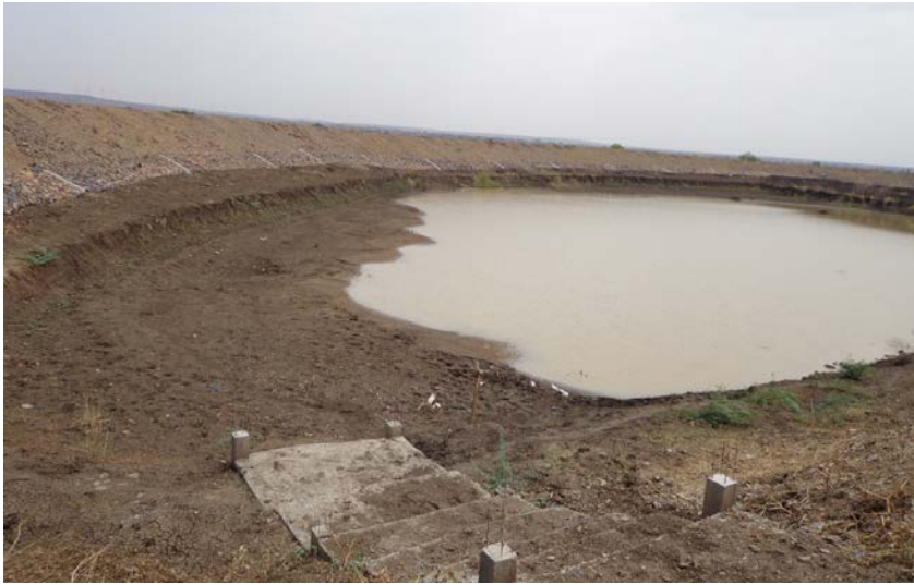
Photo 8. Desiltation of village tank under MGNREGA in Markabbinahalli
