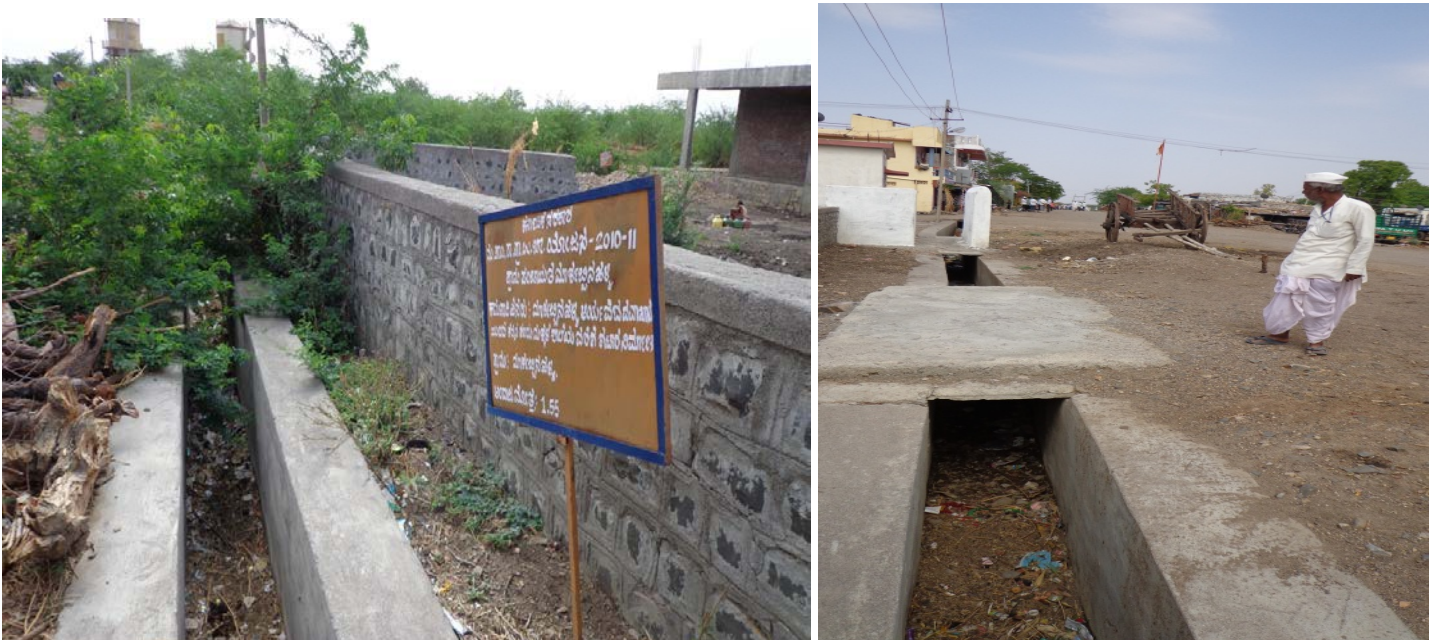
Photo 9. Drainage work under MGNREGA in Markabbinhalli
